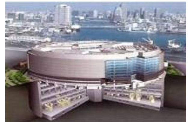
Tokyo Electric Power Shintoyosu Substation
