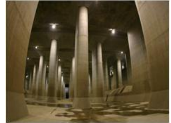
Metropolitan outer area discharge channel
