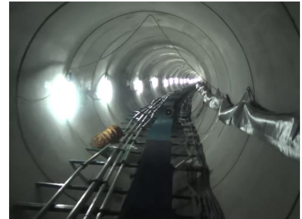
Ciliwung River discharge channel construction project
